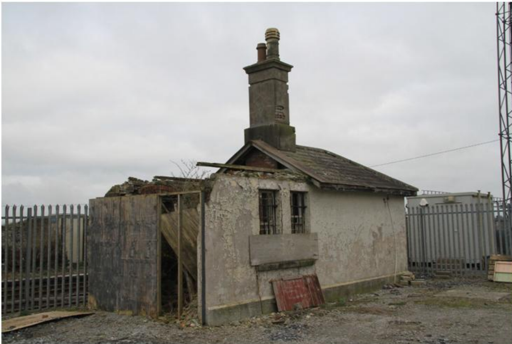
Plate 8: Single-storey building seen from south-east
