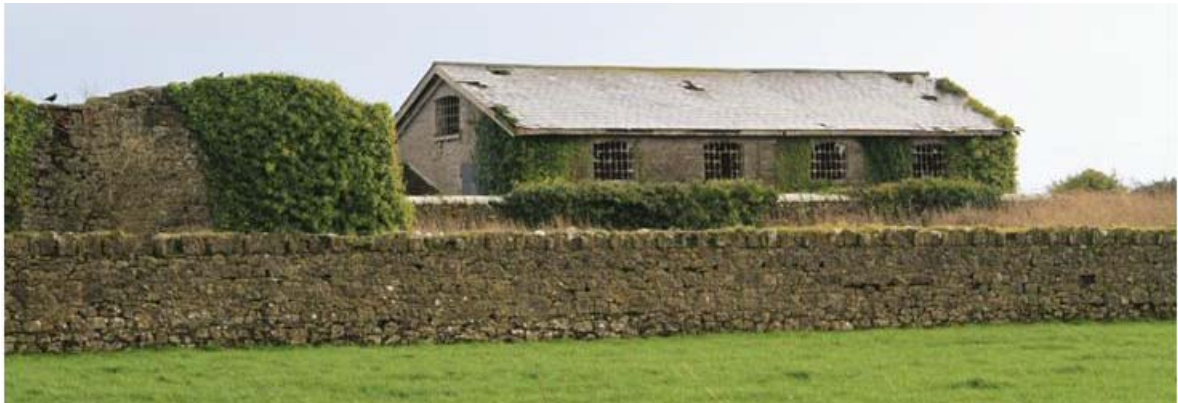
Plate 18: Western boundary wall
