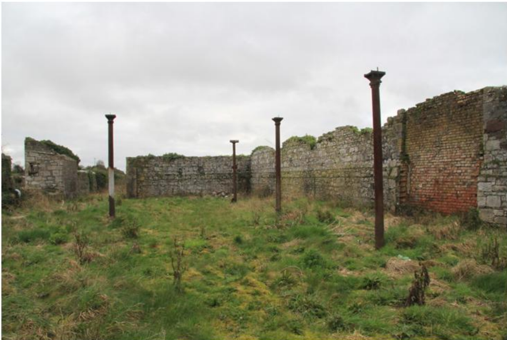
Plate 15: View southwards through former shed
