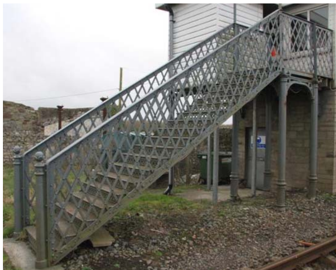
Plate 10: Stairs to signal box, taken from footbridge
