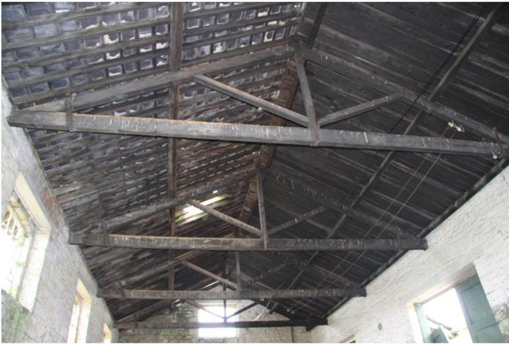
Plate 4: Internal roof structure of goods shed
