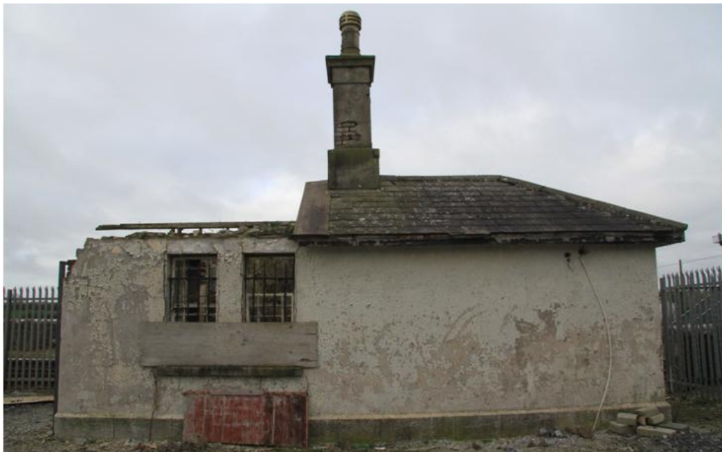
Plate 7: Eastern elevation of single-storey building
