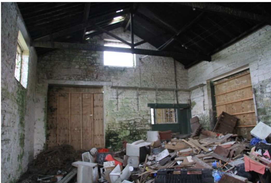
Plate 5: Interior of goods shed
