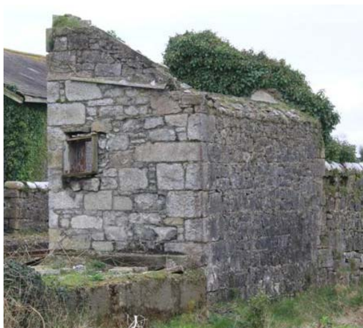
Plate 12: Shelter seen from north-west, with timber-lined ope visible
