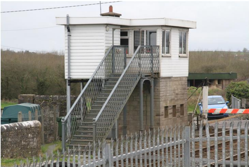
Plate 9: Signal box, with iron stairs
