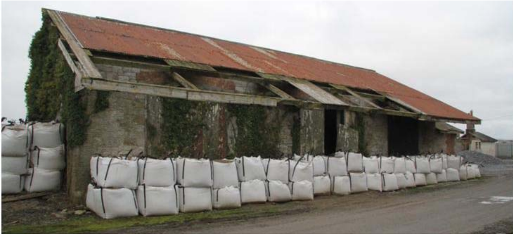
Plate 2: Goods shed seen from south-east, with canopy over loading area
